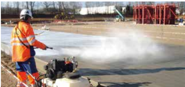
Immediate coverage or curing of concrete surfaces exposed to the elements is the most crucial step for protection of such surfaces.
