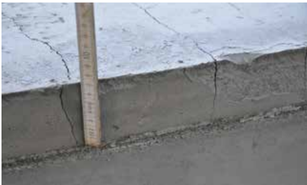
Cracks due to plastic shrinkage in a concrete pavement caused by insufficient surface protection prior to premature drying.
