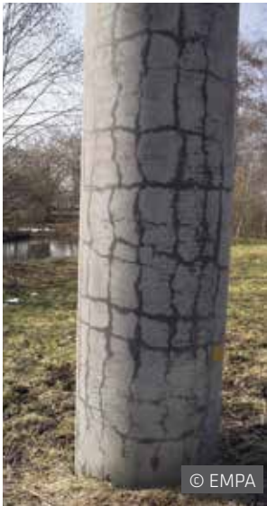
The appearance of ASR damage can be assessed very well on the drying concrete surface of this bridge pylon. Damage can appear within years or only after decades.
