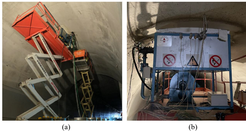
Figure 1. (a) Application of Sikacrete ® -213 F to the tunnel crown and (b) furnace for site fire resistance testing in the Panagopoula twin railway Tunnel.
