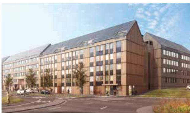
In the Swedish city of Piteå, Lindbäcks is producing standardized components in Europe's most modern modular construction facility. Modular construction is frequently used in residential building.
