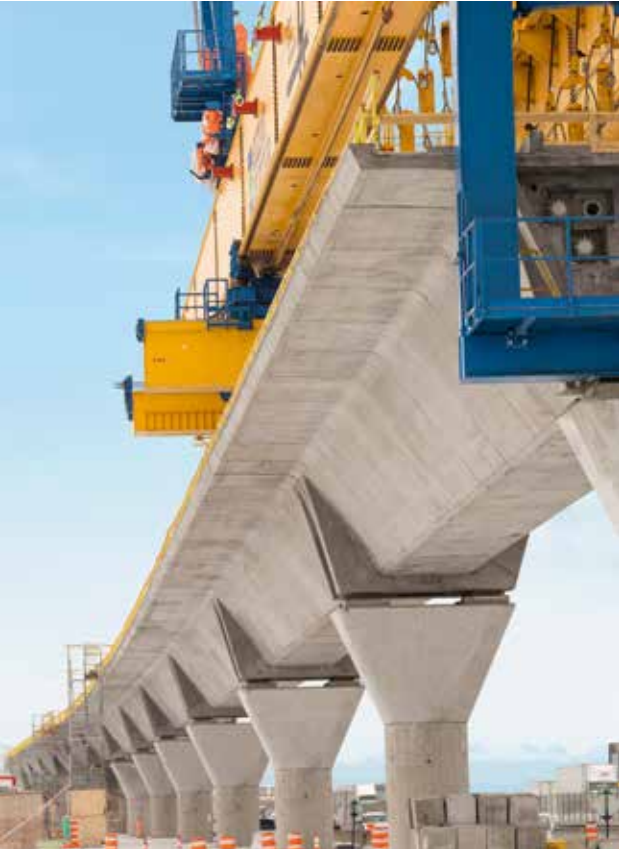
More than a third of the metro runs as an elevated railway on pillars. Concrete elements are joined together with the assistance of Sika’s high-performance structural adhesives.
