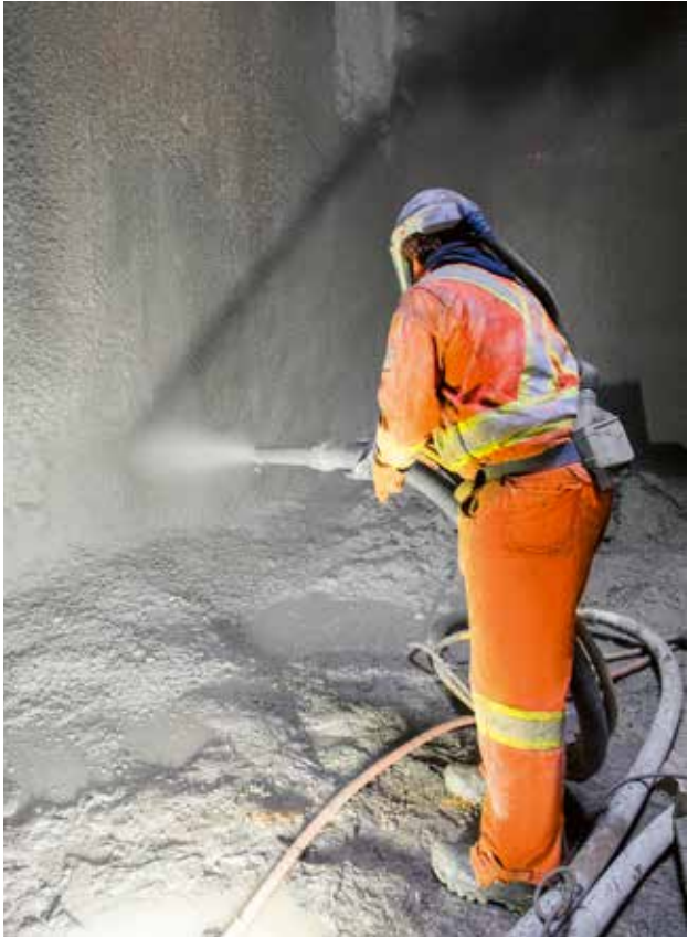
In the center of Montreal, the new light rail network is mainly built underground. Directly following excavation, the tunnel walls are secured with Sika’s shotcrete.
