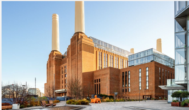
Battersea Power Station, London (UK)
